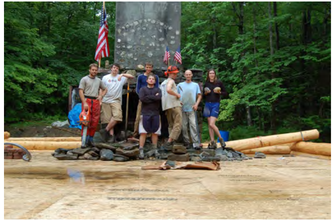
The first Crew next to the chimney.
